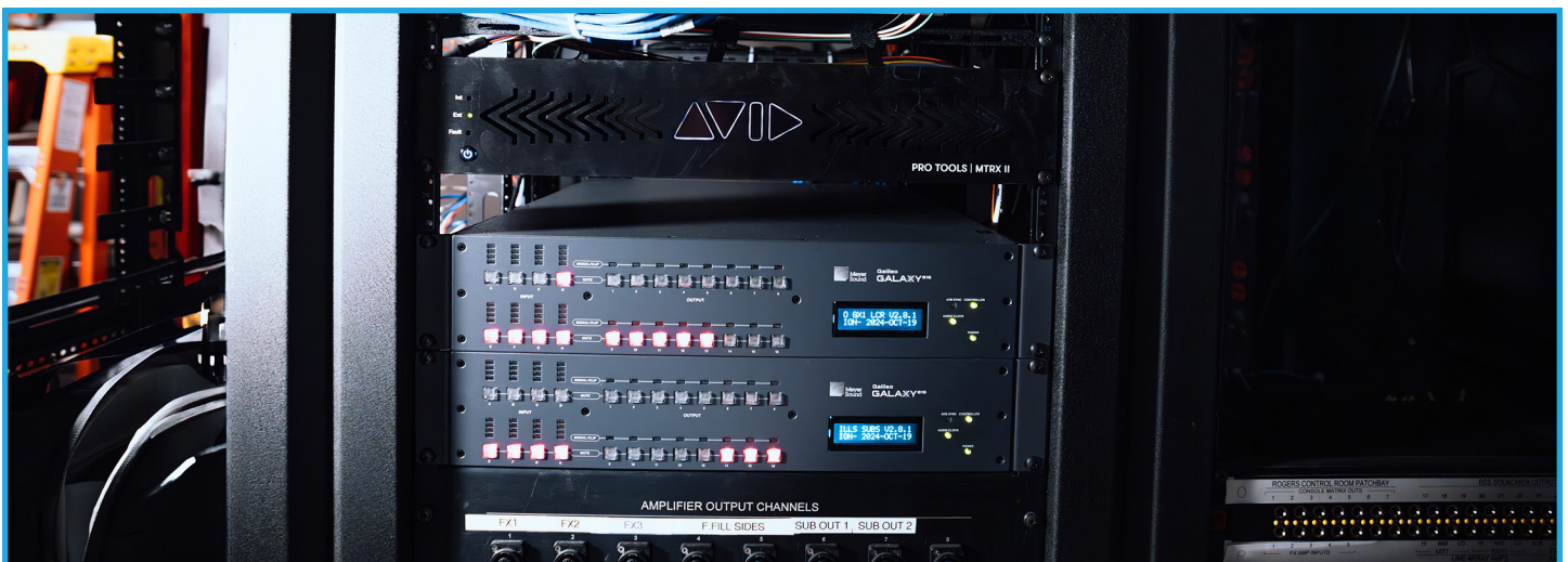
Signal processing rack with AVID MTRX II and a pair of Meyer Sound Galileo GALAXY 816 processors. Photo by Daniel Elliott.
